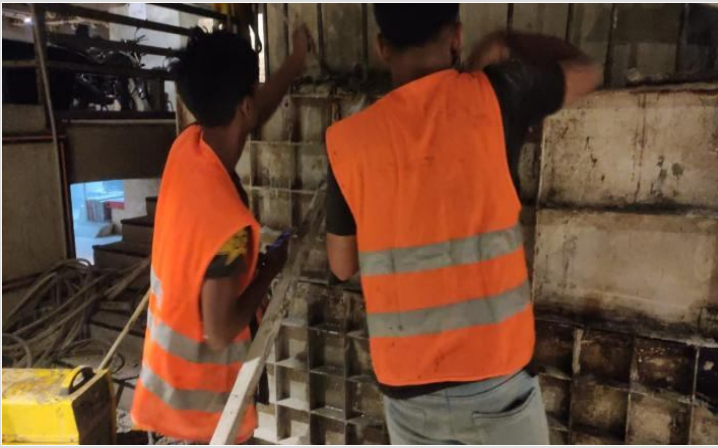
B-2-Column Retrofit shutter removing on 27-03-23
