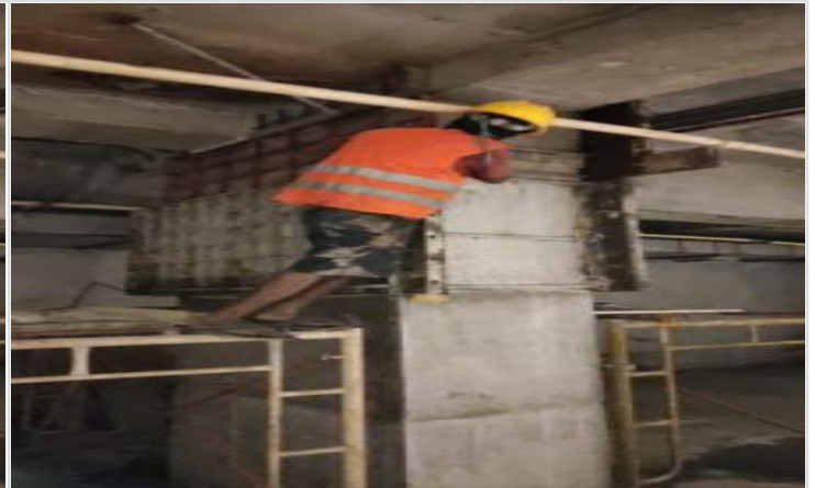
B-1-Column retrofit shuttering on 11-03-23
