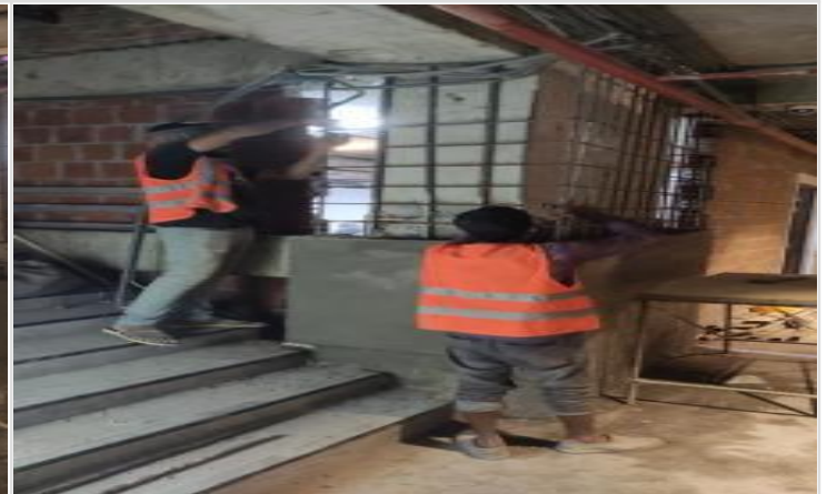
B2-Col Retrofit re-bar work on 30-03-23
