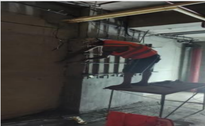
B-1-Column retrofit shuttering on 14-03-23
