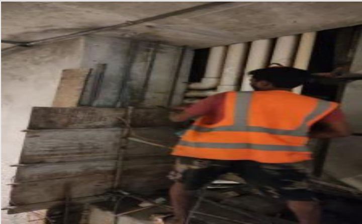
B-3-Column retrofit chipping on 20-03-23
