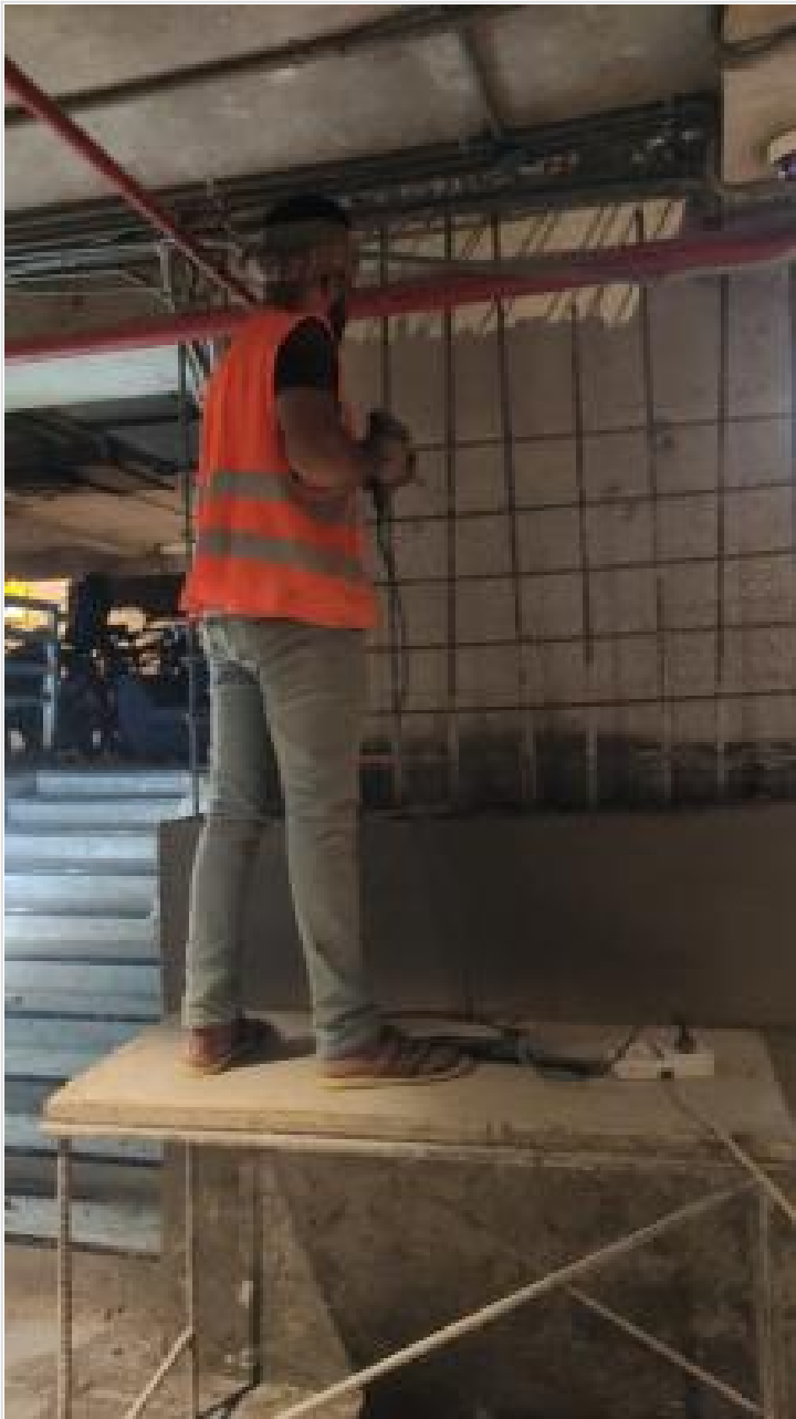
B-2-Column retrofit chipping
