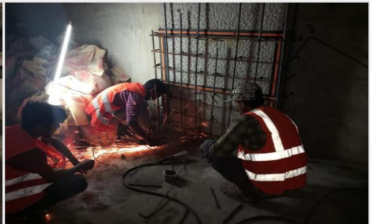
B2-Col Retrofit re-bar work on 04-03-23
