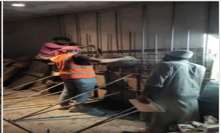
B-3-Column retrofit concreting on 22-03-23
