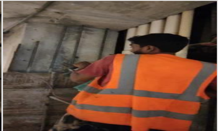
B-3-Column retrofit chipping on 20-03-23
