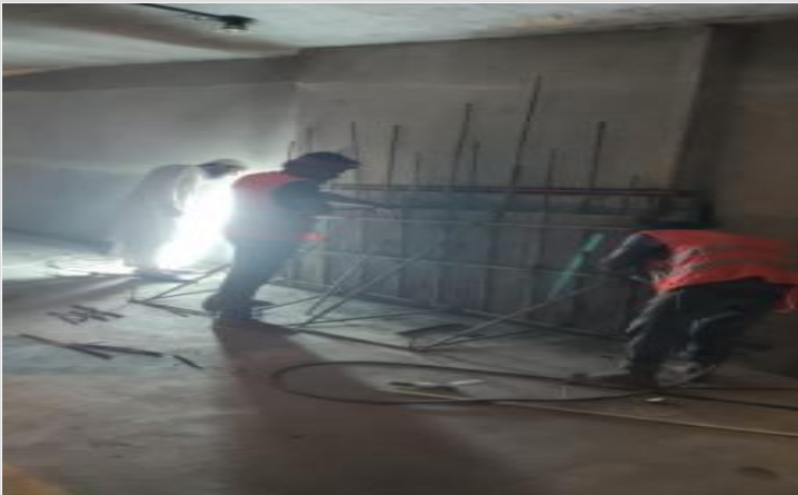
B-2 Column retrofit shuttering on 29-03-23
