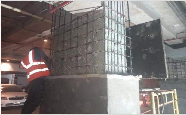
B-1-Column retrofit re-bar work on 09-03-23
