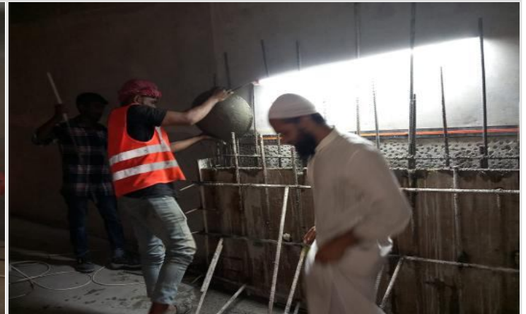
B-2-Column retrofit concreting on 29-03-23
